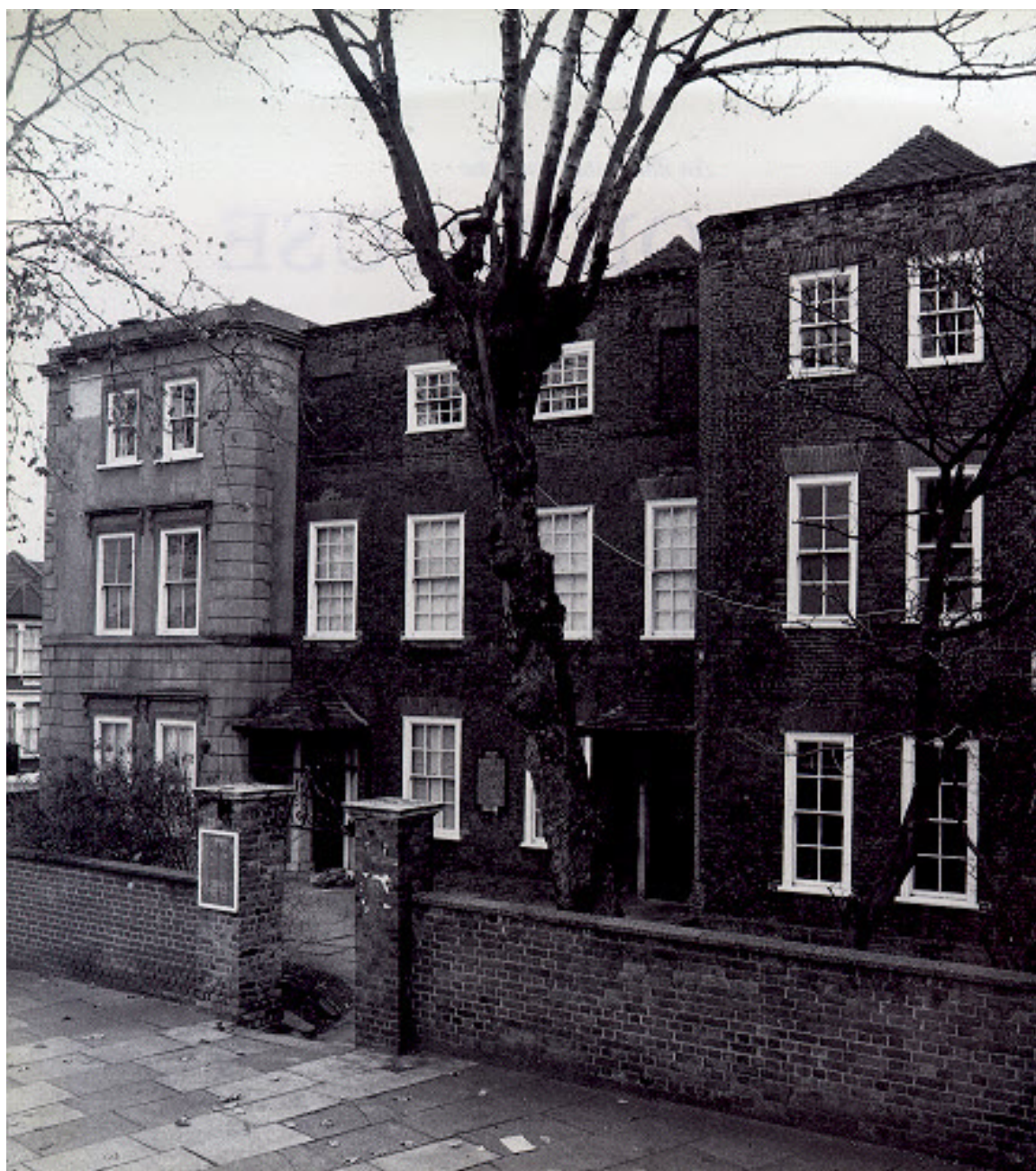
Figure 3: Sutton House in 1990 before restoration. Reproduced with the kind permission of The National Trust.
